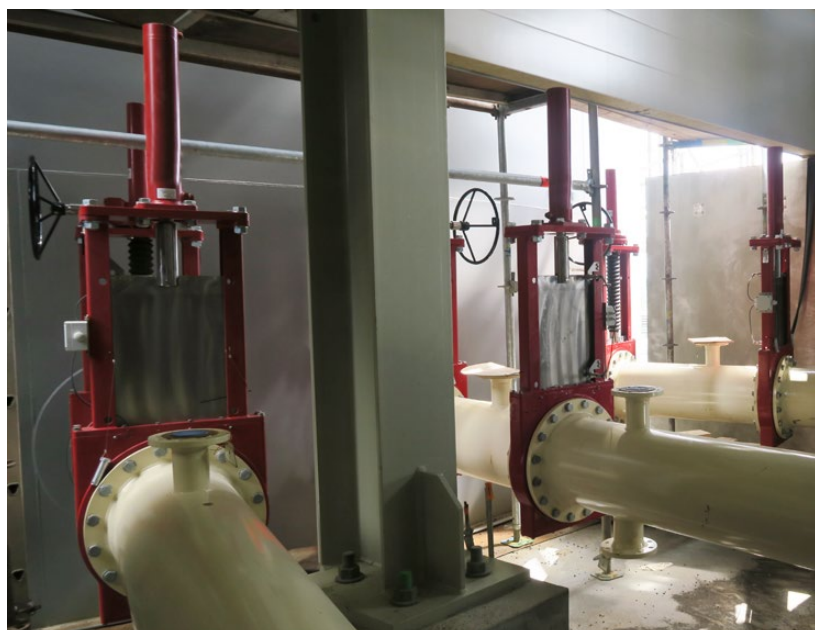
Flowrox SKW shut-off valves on the suction side of pumps in paste tanks.
